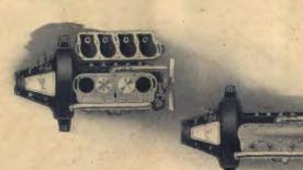
Top View of the Model T Motor, Showing Removable Cylinder Head
